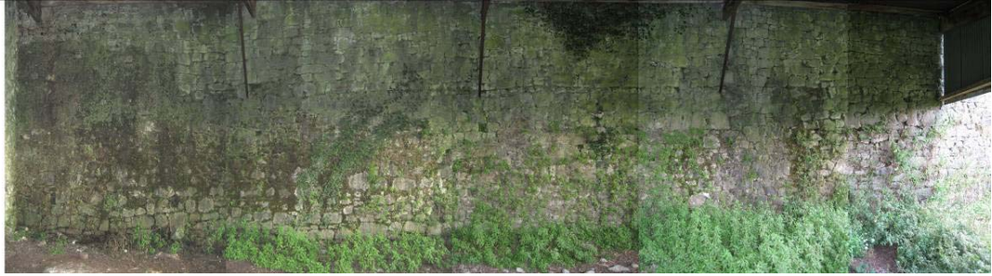
Fig. 32 Section C-2010 (Gazetteer 2.35) Mart area inside barn. Before conservation.
