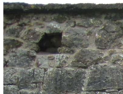
Fig 27/28 Section C-2010 (Gazetteer 2.35) North side. Rafter holes after conservation.
