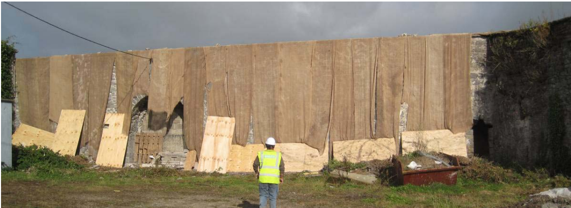
Fig. 31 Section C-2010 (Gazetteer 2.35) Mart area, east end. During conservation.
