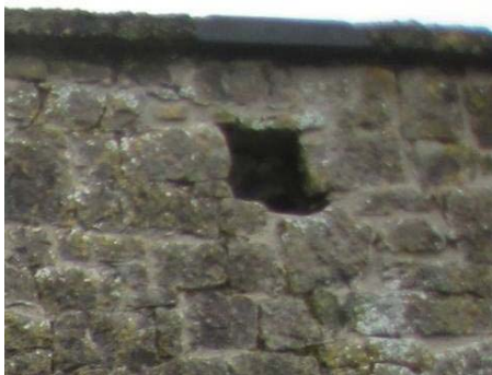
Fig 27/28 Section C-2010 (Gazetteer 2.35) North side. Rafter holes after conservation.
