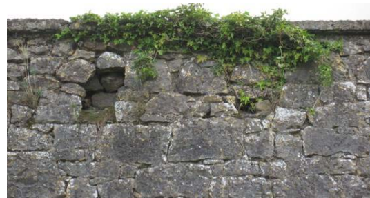
Fig 25/26 Section C-2010 (Gazetteer 2.35) North side. Loss of mortar below cap stones and around possible rafter holes. Before conservation.
