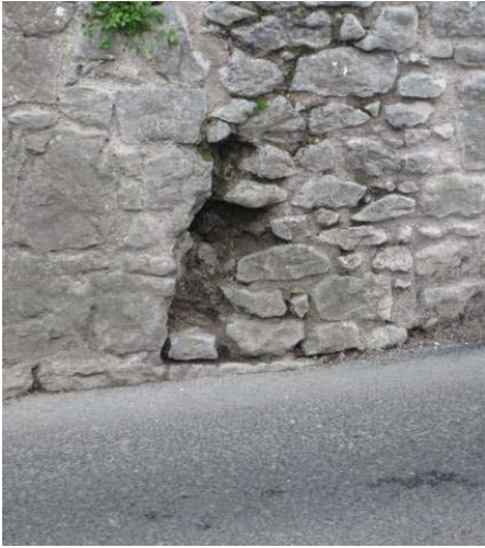
Fig. 11/12 Section A-2010 (Gazetteer 2.01) West side. Missing stones by roadway, and after conservation
