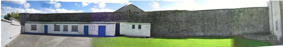
Fig. 23 Section C-2010 (Gazetteer 2.35) North side. Before conservation.
