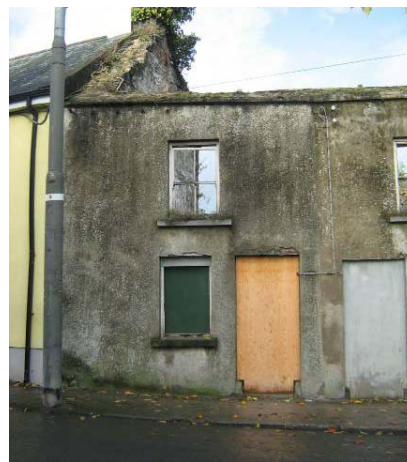
Fig. 37 View from Burke Street of wall north of east gate site.
