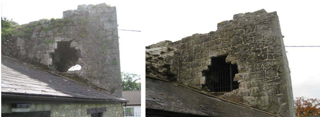
Fig. 7/8 Section A-2010 (Gazetteer 2.01) Currikeen Castle before conservation, and after.
