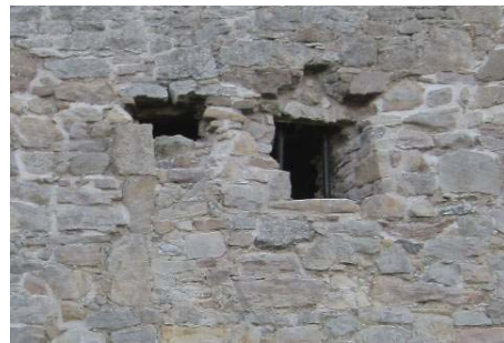
Fig 2 after pointing and with steel lintel in place
