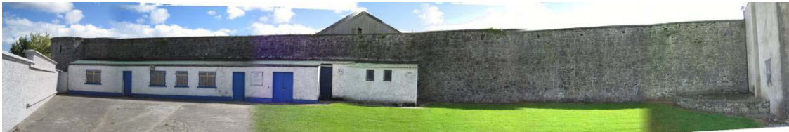
Fig. 4 View of Section C-2010 (Gazetteer 2.35)
