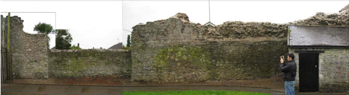
Fig. 15 Section B-2010, (Gazetteer 2.37) North side. After conservation.
