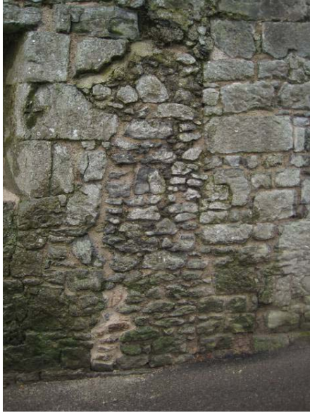
Fig. 11/12 Section A-2010 (Gazetteer 2.01) West side. Missing stones by roadway, and after conservation
