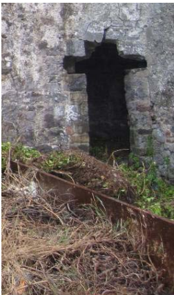
Fig. 43 Entrance to Turret (Gazetteer Section 2.34)
