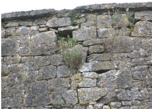
Fig 25/26 Section C-2010 (Gazetteer 2.35) North side. Loss of mortar below cap stones and around possible rafter holes. Before conservation.
