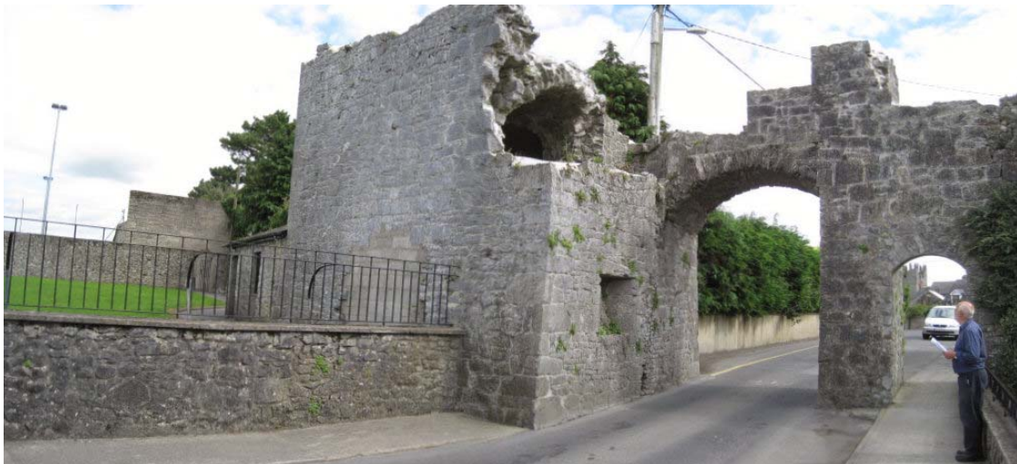
Fig. 1 View of Section A-2010 (Gazetteer 2.1)
