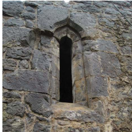
Fig.6 Window after removal of fill
